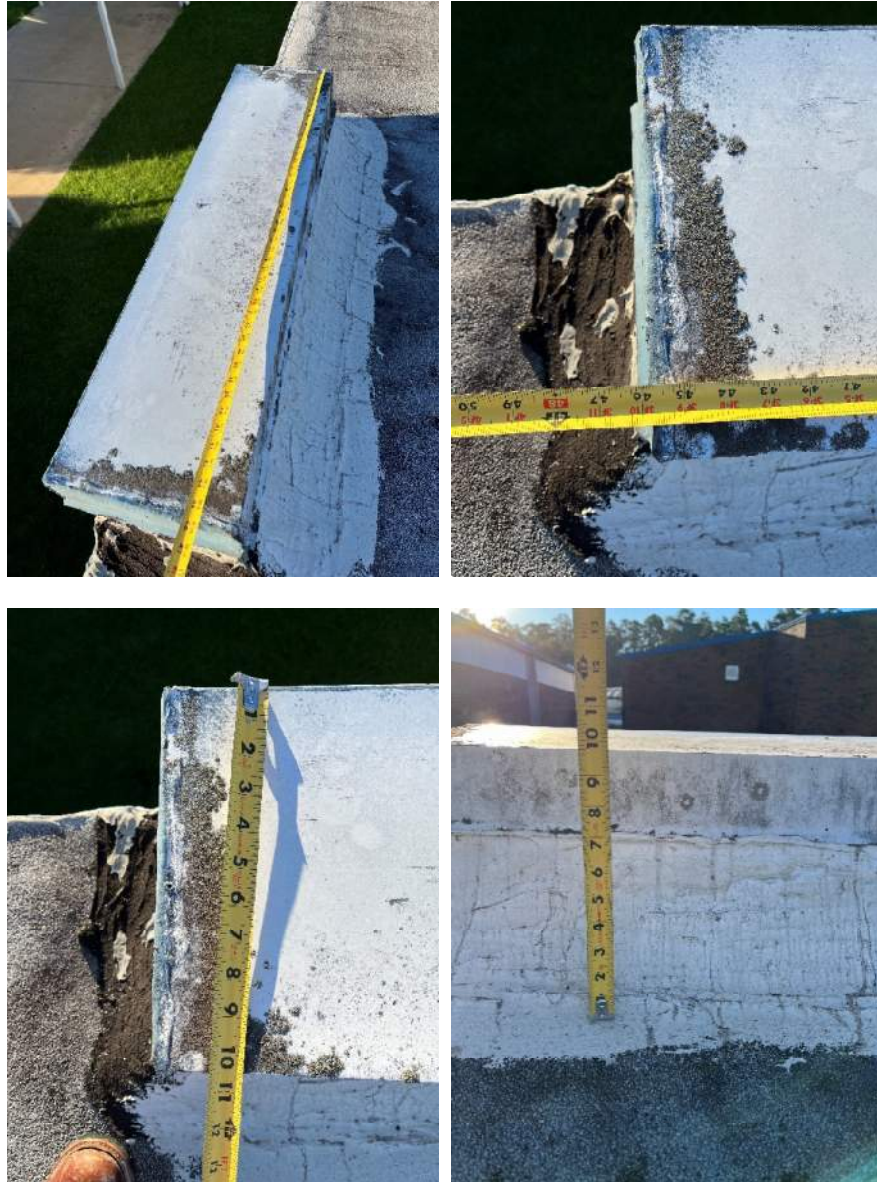
6. Roof Level – Images of concrete column parapet measurements.
