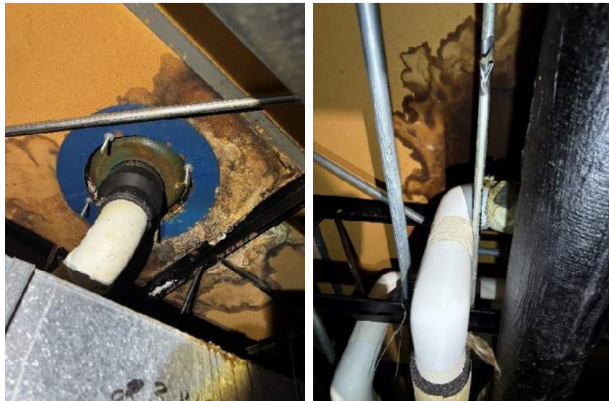
3. Level 1 – Stains on existing formboard – some at existing roof drain locations.
